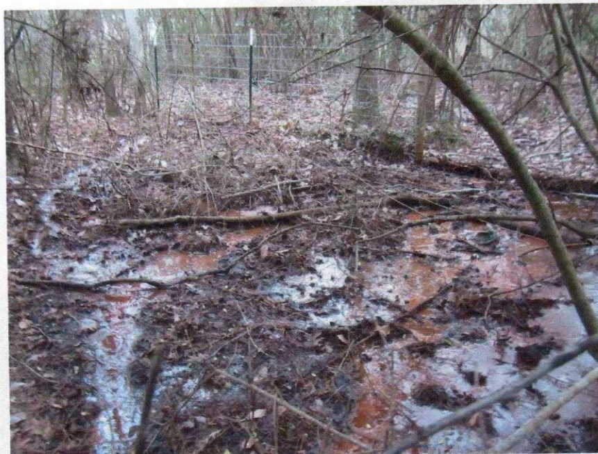
Photo 10: View of the flow from the seepage noted in photo 9. This photo was taken from the right side of the dam at the edge of the fence line, facing the upstream direction of the seepage flow (southwest).
