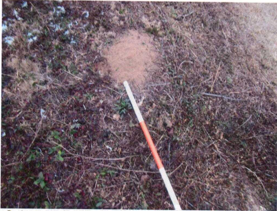
Photo 3: An example of the anthills noted in the dam crest. This example was found on the left side of the dam, facing northwest.
