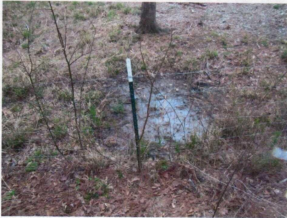
Photo 12: View of an area of standing water, on the right side of the downstream toe, facing downstream (south).
