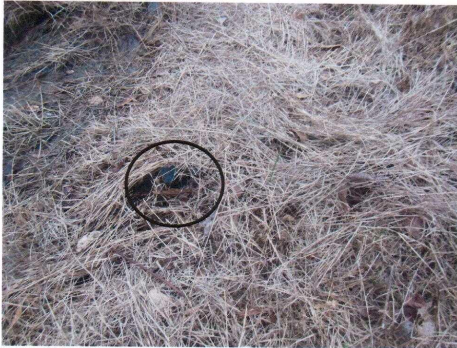
Photo 7: An example of the root balls (circled) and stumps left in the upstream slope. This photo was taken on the right side of the dam, facing northeast.
